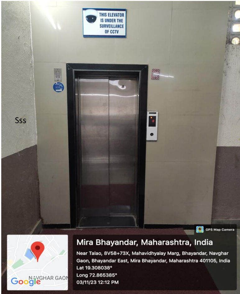
A Modern Elevator for Divyanjans in the Campus
